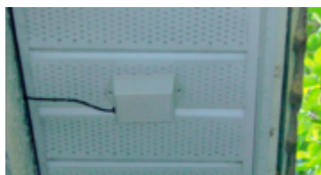
Outdoor Humidity/Temp Sensor installed under eave
